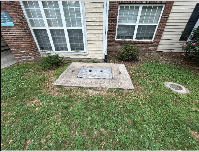
67. Sanitary sewer station
