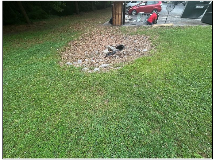
68. Stormwater management drainage pipe
