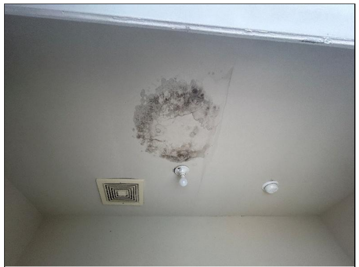
42. Microbial growth in pool pump room
